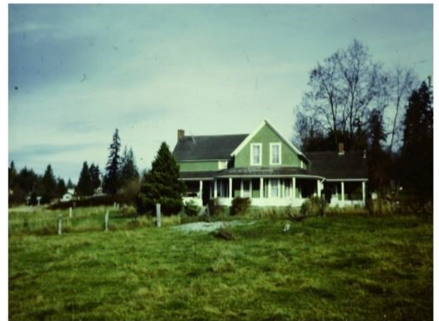
The Beckstrom House
