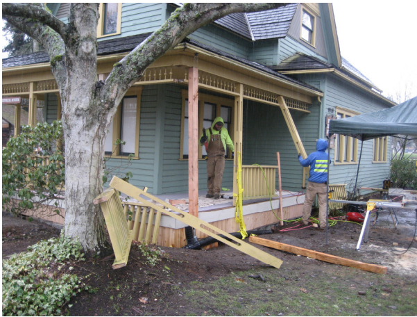
Rebuilding the Hannan House Porch
